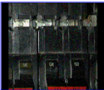
FIGURE 5 - THE ENDS OF THE SCREWS HOLDING THE STAB SOCKET PLATES ARE VISIBLE BETWEEN THE TWO ROWS OF BREAKERS. THIS IDENTIFIES IT AS A PANEL OF THE TYPE SHOWN IN FIGURE 2-C [Click for larger image]
