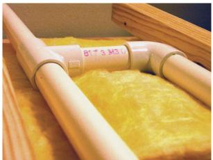
Photo: During this inspection, the primary and secondary drains were discovered tied together, negating much of the value of a second drain. Photo TS Hart.
