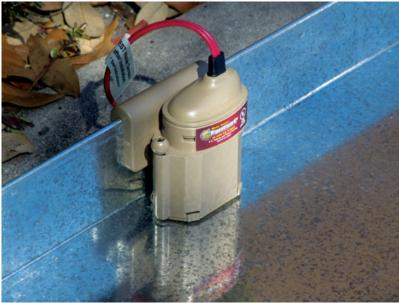
Photo: The water sensor seen in the photo attaches to the side of the auxiliary drain pan and will shut off the cooling equipment as the pan fills with water. Photo courtesy Resource Conservation Technologies, makers of AquaGuard brand HVAC accessories.
