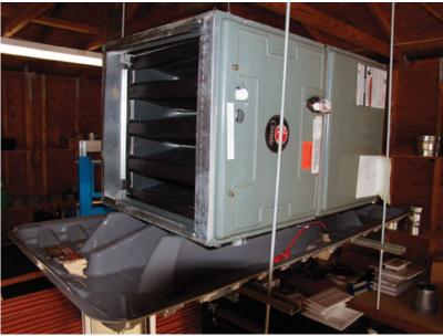
Photo: Manufactured auxiliary drain pans, like the one in the photo, hold the air handler or furnace above the overflowing condensate. This is important as it can prevent damage to the equipment and make the pan easier to clean. Photo courtesy Resource Conservation Technologies, makers of AquaGuard brand HVAC accessories.
